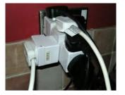
There must only ever be one adapter inserted into a mains socket and there must never be an adapter linked to another adapter.
